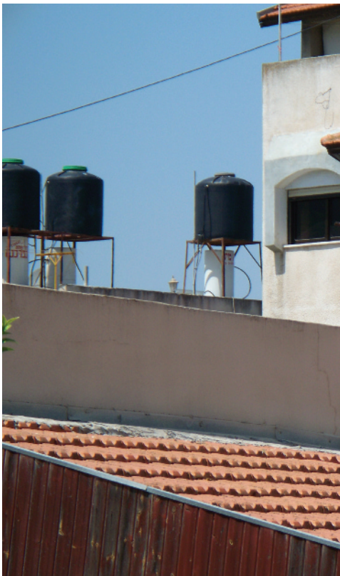
FIGURE OCCUPATIONS 2 Solar water heaters mounted on a roof.
