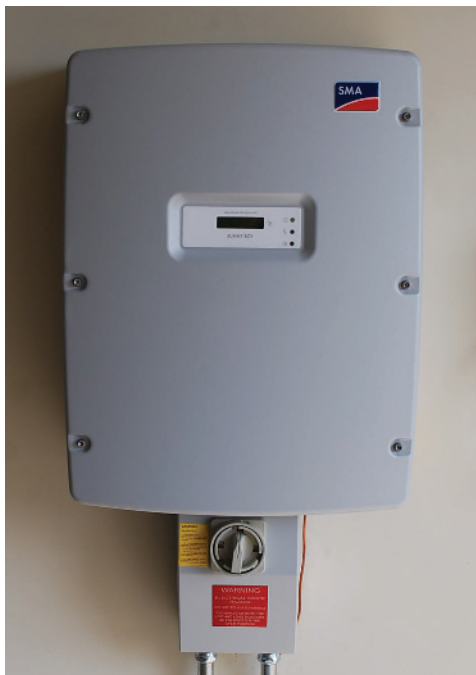
FIGURE OCCUPATIONS 5 Inverter changes the direct current produced by the solar cells into alternating current.
